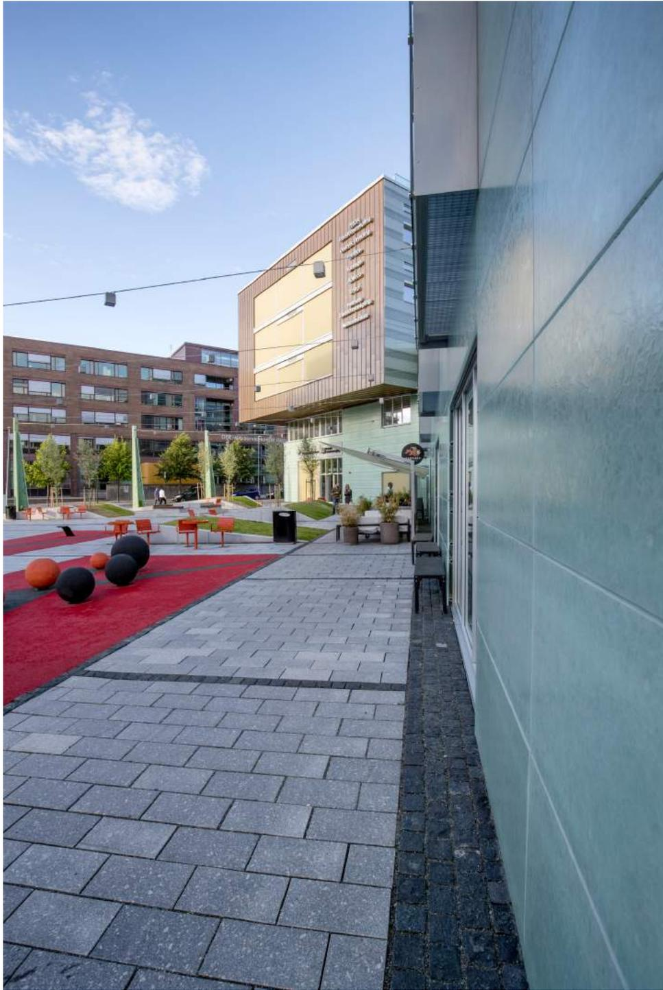
The material offers a new and sustainable circular economy ethic, whereby the entire contents are sourced and upcycled from trade waste glass and can be locally recycled by glass processors at the end of a long life. The material is heavily durable, offering true performance and tested certification as well as suited to both hot and cold climates, strong against vandalism, impervious to staining and almost self-cleaning in its finish.
