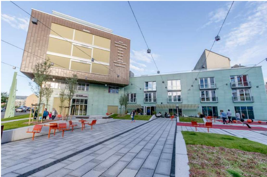
The building is clad with a range of systems from curtain walling to rainscreen, however the near 400M2 rainscreen areas are applied with Magna Glaskeramik in type Jade Patinated, thickness 21mm panels with 10mm open joints between panels and a Fischer ACT Aluminium rail under-construction method to hang the cladding back to the concrete structural frame.
